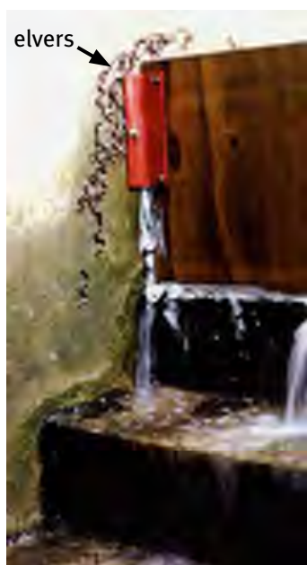
Eels have the ability to ascend damp vertical surfaces (left), but passage is far more successful if we provide ramps with climbing substrate, like this one on Mallemort Dam in France (right). Alex Haro
