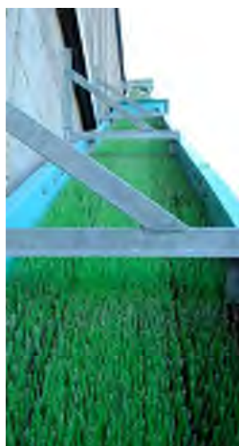
Eels have the ability to ascend damp vertical surfaces (left), but passage is far more successful if we provide ramps with climbing substrate, like this one on Mallemort Dam in France (right). Alex Haro
